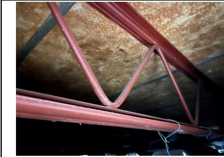
5. View above the ceiling in Room 129.
