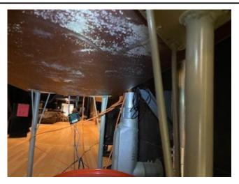
Visible mold was observed under a table on the Auditorium Stage near the ELECTRO CONTROL panel.
