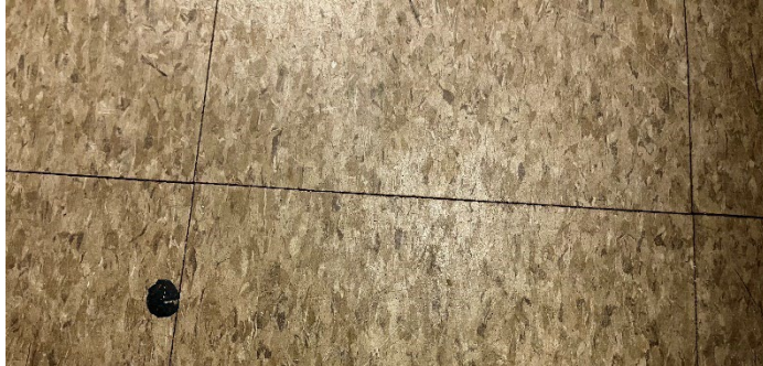
13. HA 13-Non asbestos containing light brown 12" x 12" floor tile with marble pattern.
