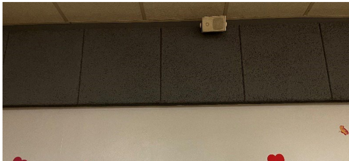
44. HA 44-Non asbestos containing brown sound boards.
