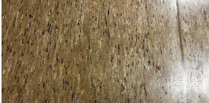
43. HA 43-Non asbestos containing tan linoleum with brown and white streaks and associated mastic.
